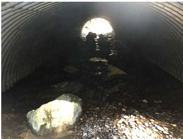
Looking through from outlet
