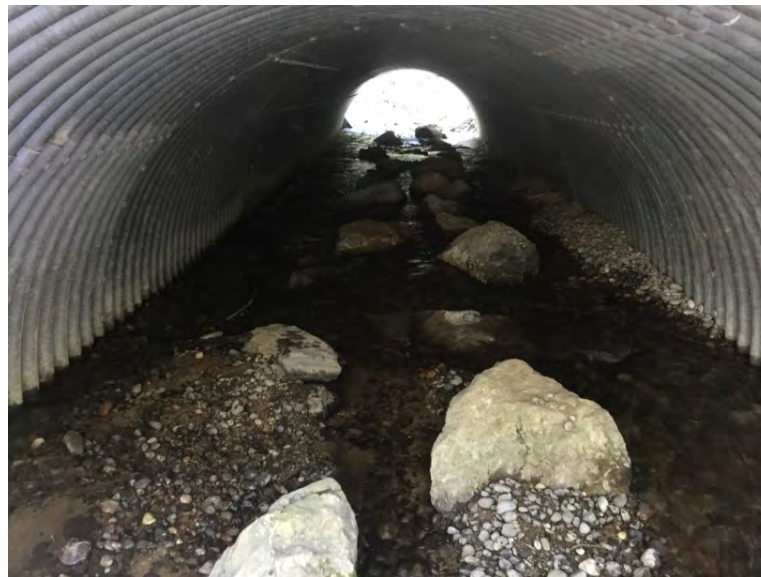
Looking through from inlet
